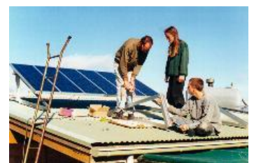
Helping Dad install the new solar panels. Thomas, now 17, monitors the system.
